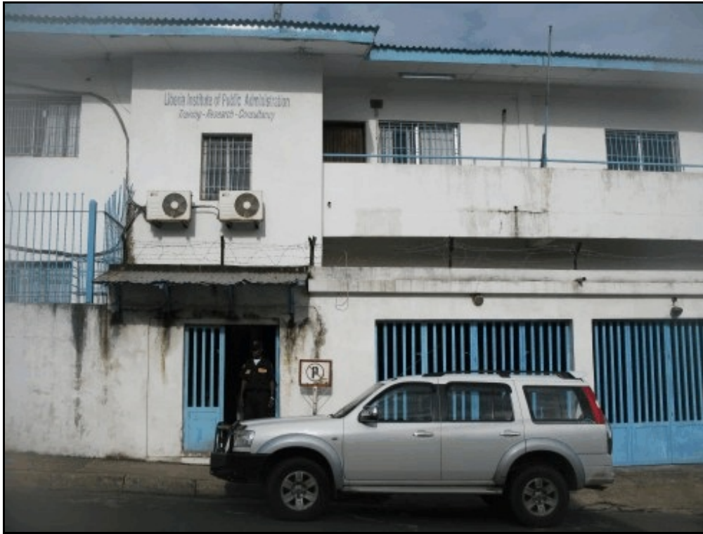
Front view of my office building.
