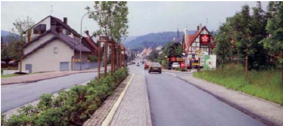
Median with plants and trees. Atlanta Regional Commission, Context Sensitive Street Design 17 (2001), at http://atlantaregional.com/qualitygrowth/Context_Sensitive_TOOL.PDF .
